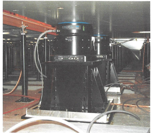
STACIS® 2100 on a "riser" installed under a TMC platform in a 36" tall raised floor
